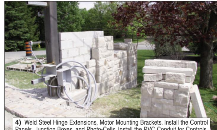
4) Weld Steel Hinge Extensions, Motor Mounting Brackets. Install the Control Panels, Junction Boxes, and Photo-Cells. Install the PVC Conduit for Controls, Safety Equipment, Lights, and spares for future use.
