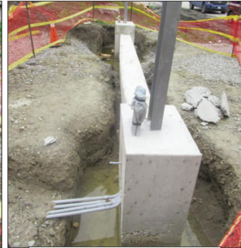
3) After concrete has cured, remove the Form Work, Clean Up and Back Fill.
