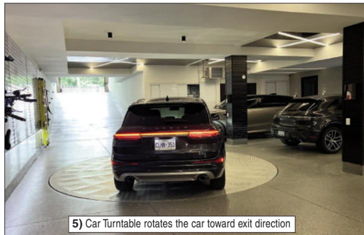
5) Car Turntable rotates the car toward exit direction
