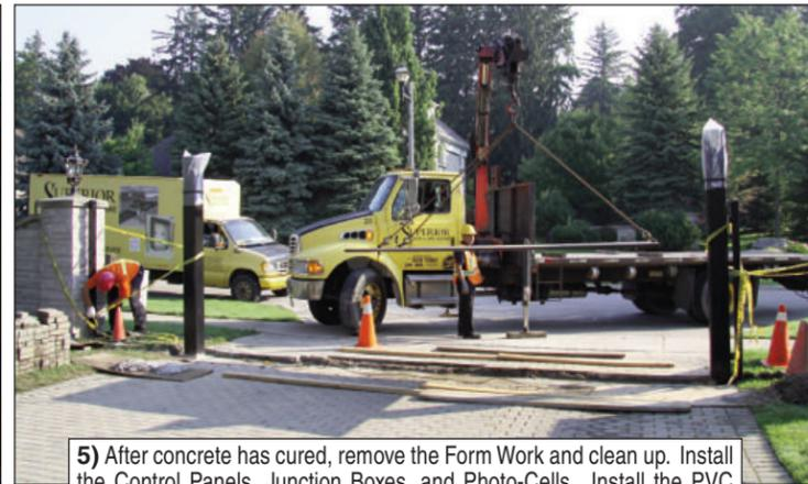
5) After concrete has cured, remove the Form Work and clean up. Install the Control Panels, Junction Boxes, and Photo-Cells. Install the PVC Conduit for Controls, Safety Equipment Lights, and spares for future use.
