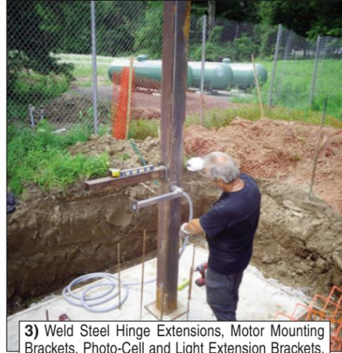
3) Weld Steel Hinge Extensions, Motor Mounting Brackets, Photo-Cell and Light Extension Brackets. Install PVC Conduit for Power, Controls, Safety Equipment and Communication.
