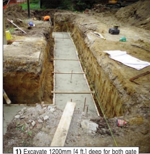
1) Excavate 1200mm [4 ft.] deep for both gate posts and across the driveway. Pour 200mm [8"] Concrete Foundation Base
