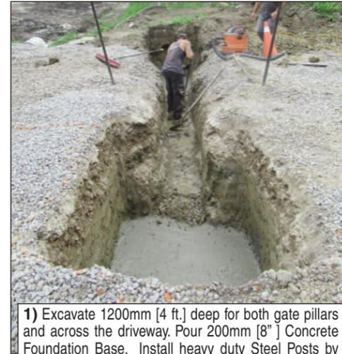
1) Excavate 1200mm [4 ft.] deep for both gate pillars and across the driveway. Pour 200mm [8"] Concrete Foundation Base. Install heavy duty Steel Posts by bolting to the Concrete Foundation base to support the Stone Pillars.
