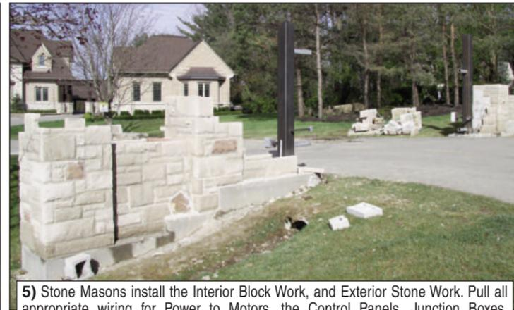
5) Stone Masons install the Interior Block Work, and Exterior Stone Work. Pull all appropriate wiring for Power to Motors, the Control Panels, Junction Boxes, Including Lights, Vehicle Sensing Loops, Photo-Cells, and Cellular Phone Systems.
