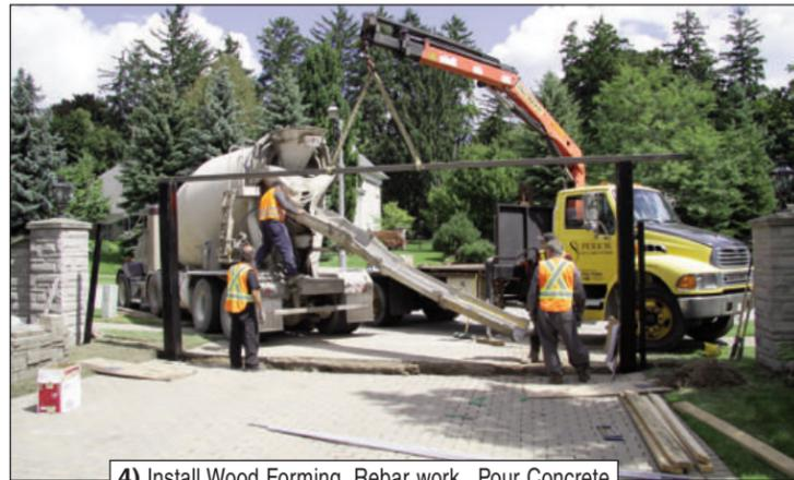
4) Install Wood Forming, Rebar work. Pour Concrete as required to suit Asphalt or Stone Driveway Finishes.
