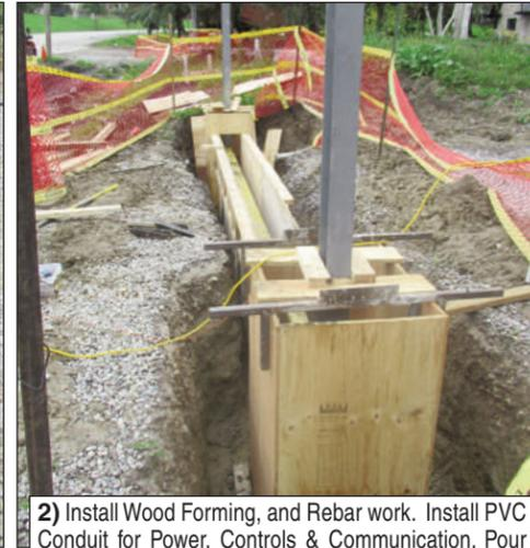
2) Install Wood Forming, and Rebar work. Install PVC Conduit for Power, Controls & Communication. Pour Concrete as required to suit Asphalt or Stone Driveway Finishes
