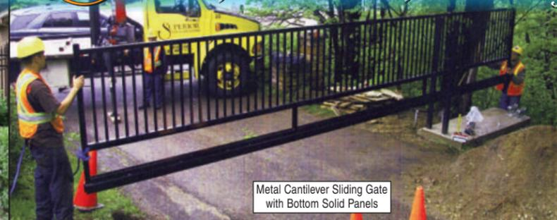
Metal Cantilever Sliding Gate with Bottom Solid Panels
