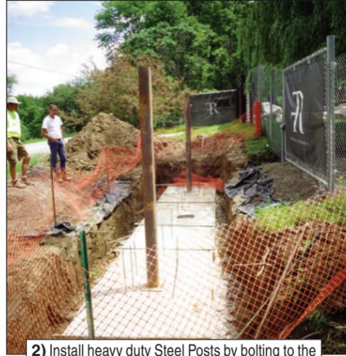
2) Install heavy duty Steel Posts by bolting to the Concrete Foundation Base to support the Heavy Gates.
